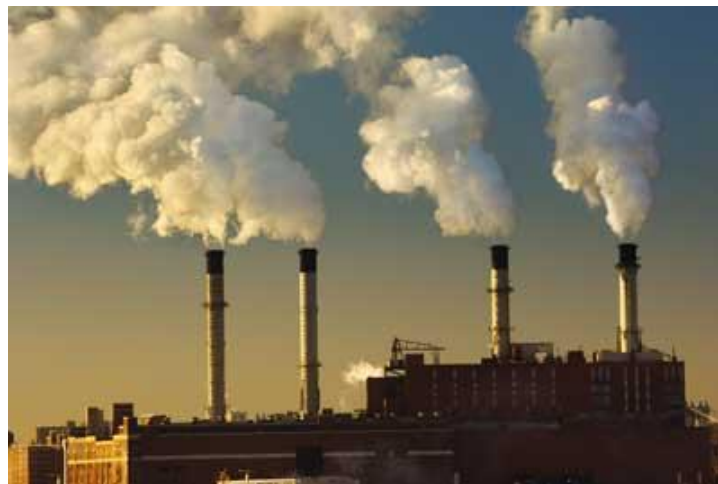
Figure 5: Coal-fired Power Plant in Pennsylvania
