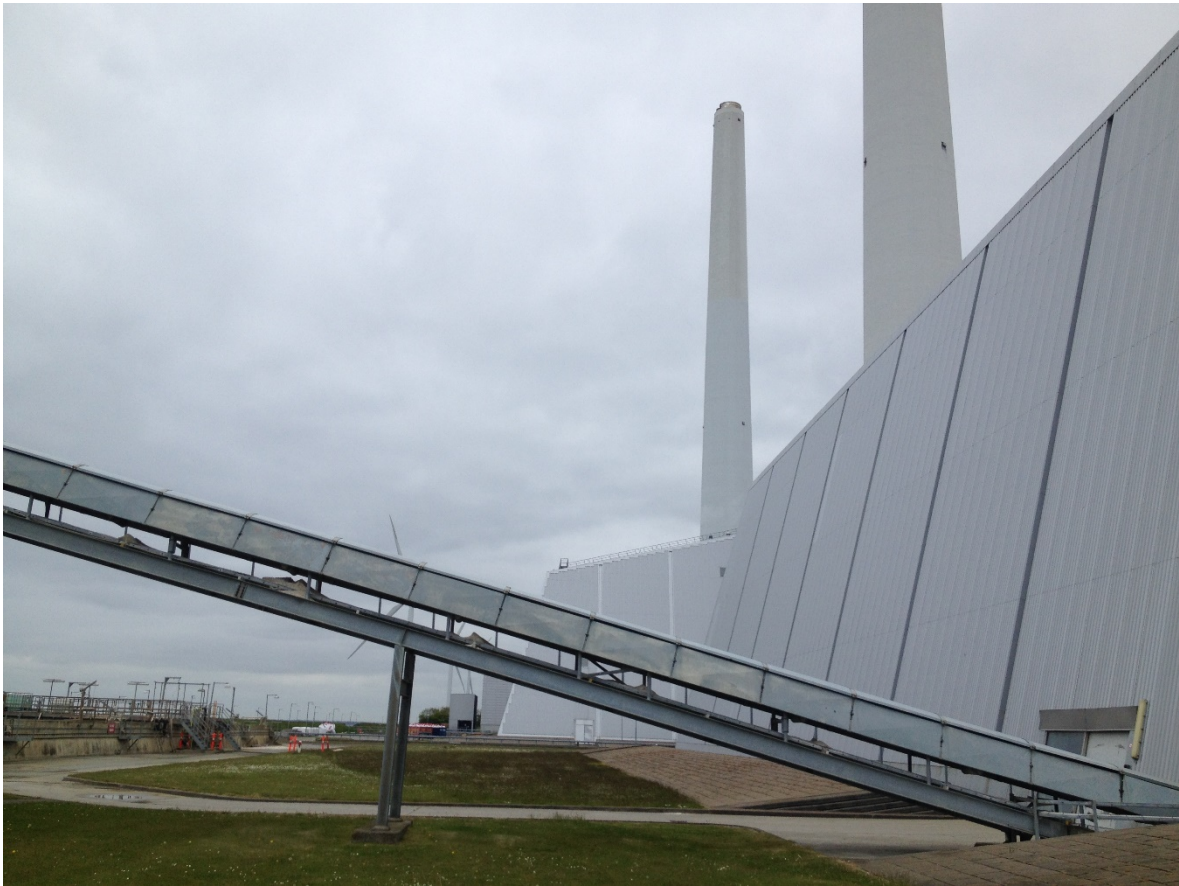
[2] Denmark, Copenhagen, Dong Energy power plant - belt conveyor
