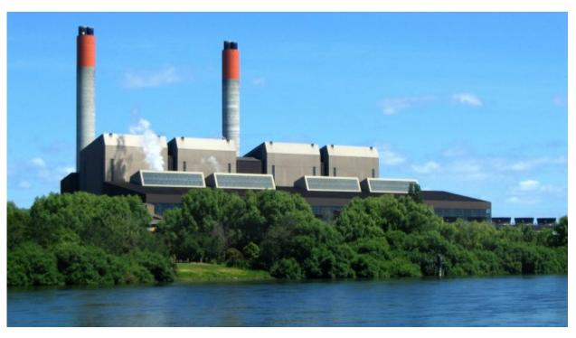
The Huntly power station is the largest thermal power plant in New Zealand. Based on the banks of the Waikato River, Huntly is owned and operated by Genesis Energy, one of the larger energy companies in New Zealand. When running at full capacity, the plant is able to supply 31% of New Zealand's electricity needs. The plant consists of four coal and two gas fired turbines. Auckland is the main market for electricity produced at Huntly.
