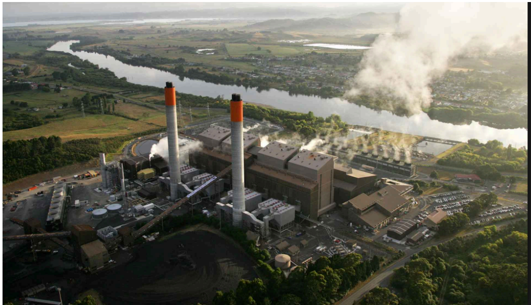
Figure 1: Overview of Huntly Power Station
