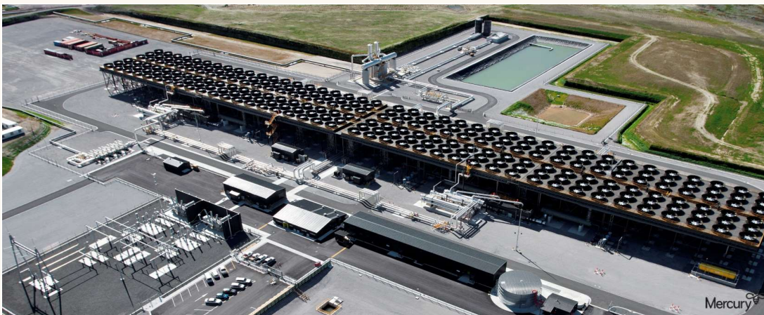
Ngatamariki 82 MWe Geothermal Power Station (Mercury NZ / Tauhara North No.2 Trust)
