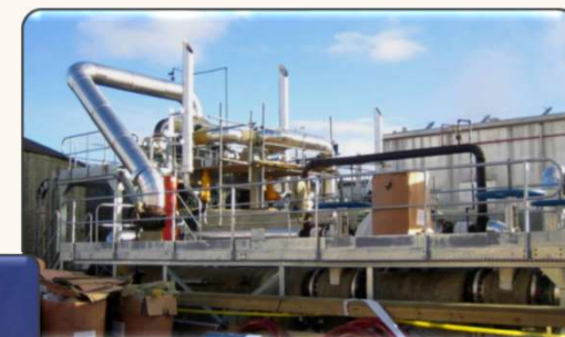
Heat Plant (during construction)
