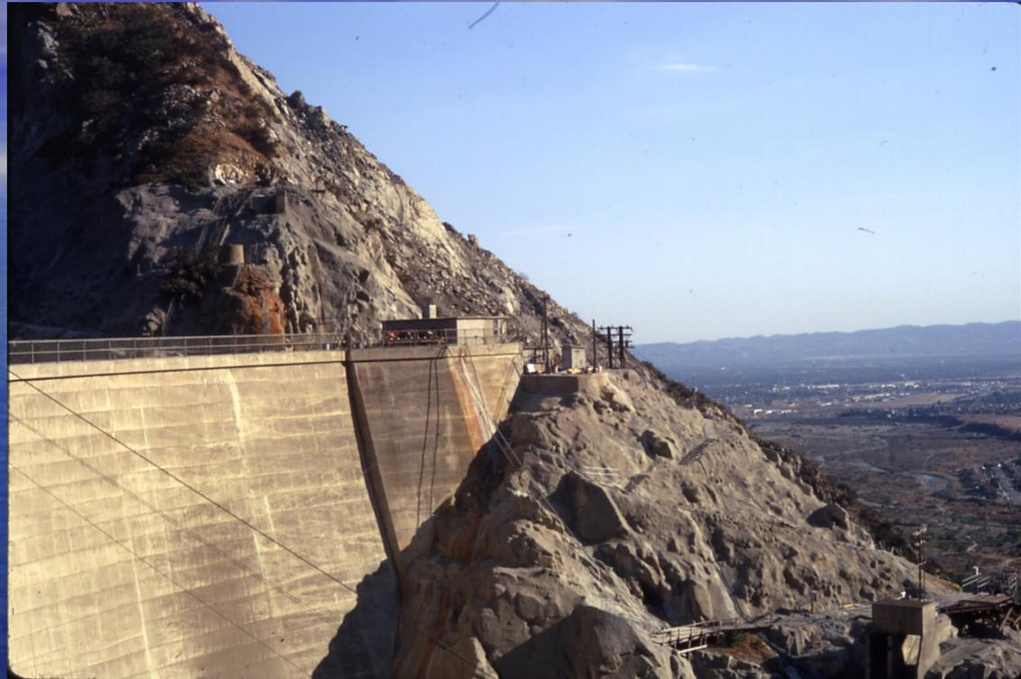
Dick served as a consultant on Pacoima arch dam; which was the world's highest dam until Hoover Dam. It was founded on extremely fractured rock, which recorded an acceleration of 1.3g in the 1971 San Fernando earthquake.
