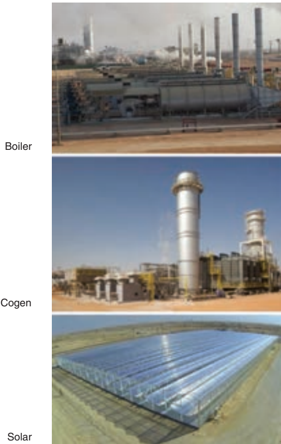
Fig. 1—The three methods of steam generation.
